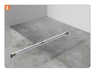
The subfloor must be clean and dry and if necessary, smoothed with a self-levelling compound to give an even surface.
