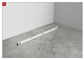
The subfloor must be clean and dry and if necessary, smoothed with a self-levelling compound to give an even surface.
